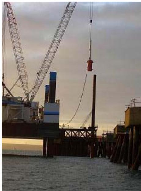
Figure 3.1 Impact pile driver being prepared to be placed onto pile
