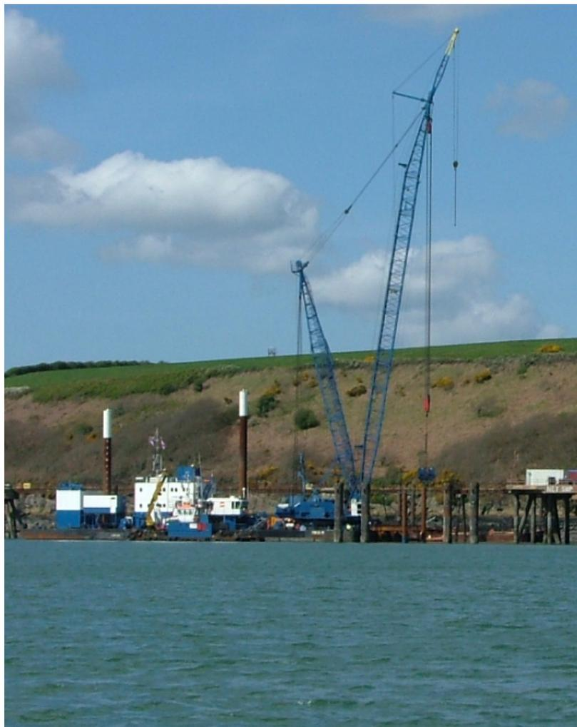
Figure 3.2 Vibratory pile driving in progress
