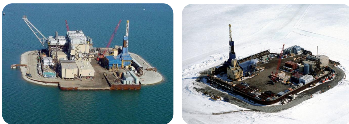
Figure 5.16 Artificial drilling and production island Northstar in open water (left, from www.wikipedia.org ) and icebound (right, from oilrig-photos.com )
