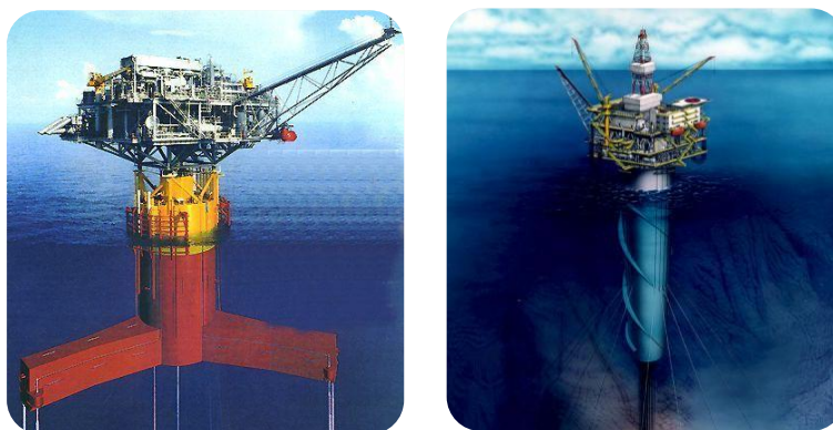
Figure 5.30 Illustration of a tension-leg platform (left) and a spar platform (right)
