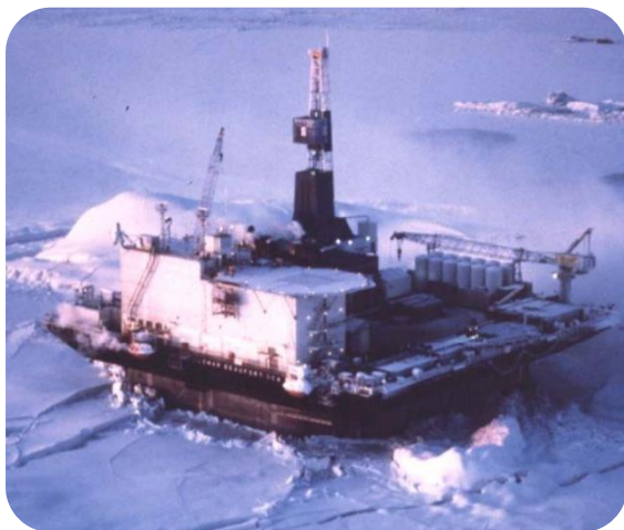
Figure 5.18 Concrete island drilling system Glomar Beaufort 1 (aka Orlan ) under severe ice pressure conditions (left) and diagram of its structural elements (right). From www.precastdesign.com
