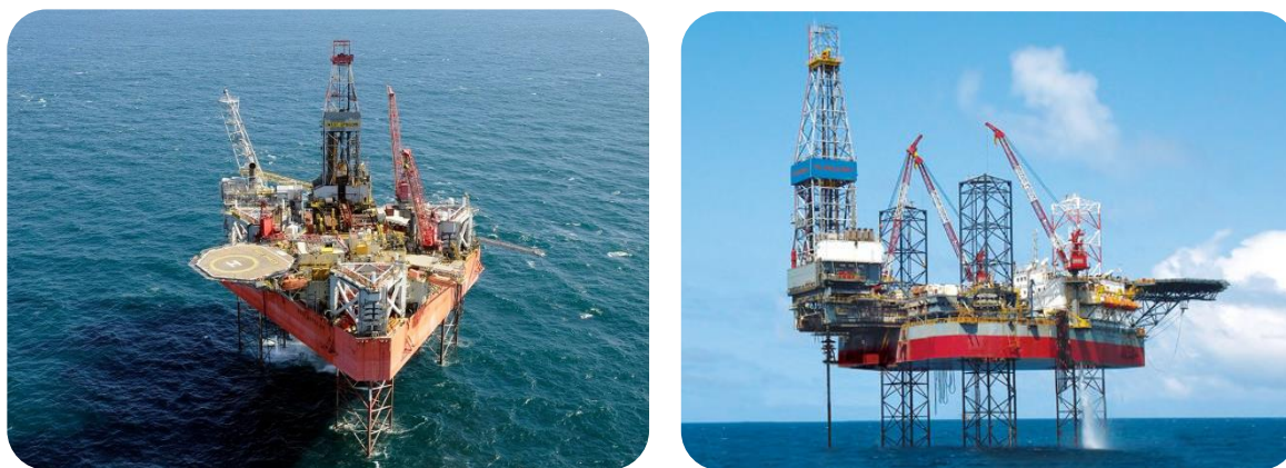
Figure 5.15 Plan view (left, from www.ogj.com ) and lateral view (right, from www.pvdrilling.com ) of two jack-up drilling rigs.
