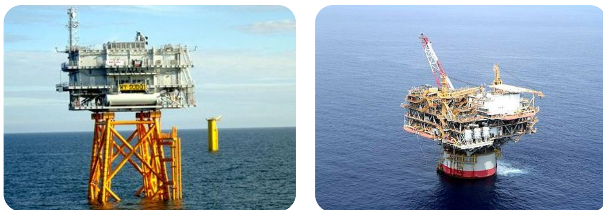
Figure 5.14 Conventional jacket (left) and spar (right) fixed drilling platforms
